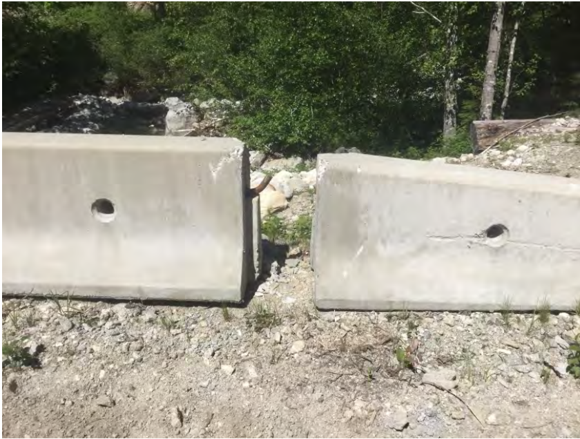
Downstream right approach barrier
