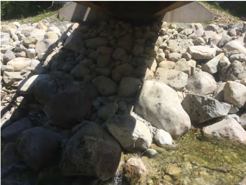
Right Bank Abutment when facing downstream
