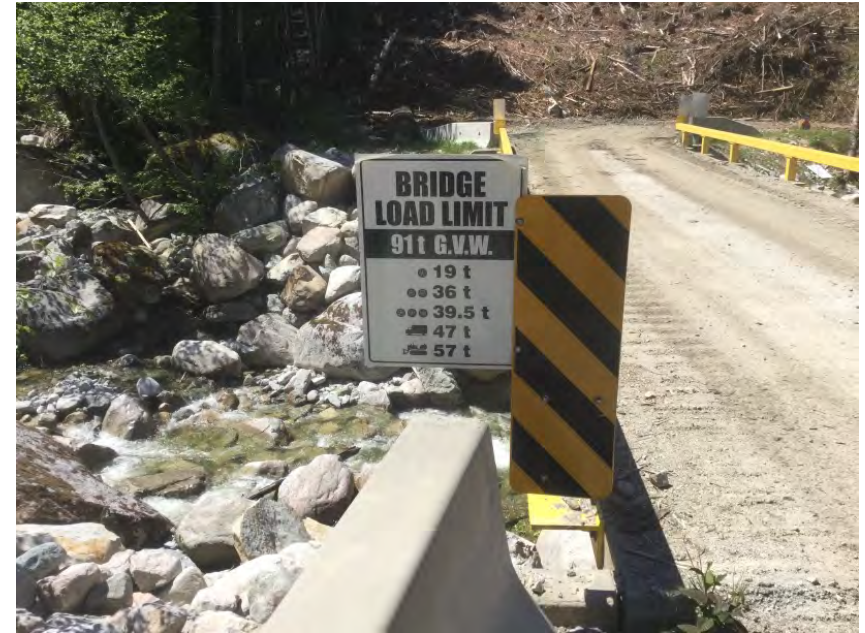
Load Rating Sign
