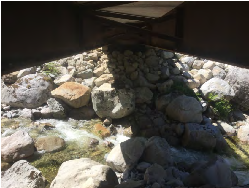
Left Bank Abutment when facing downstream
