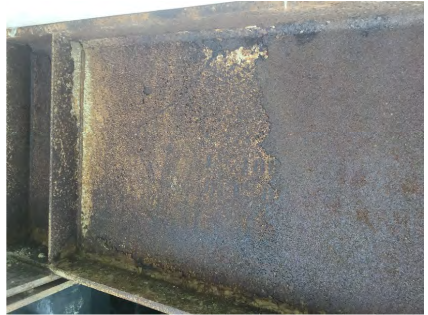
Girders appear older than abutments and deck
